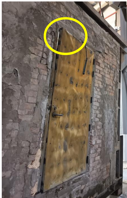
Figure 12: The exposed face after the test.
