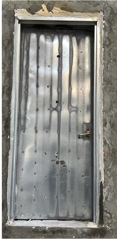
Figure 13: The un-exposed face after the test.
